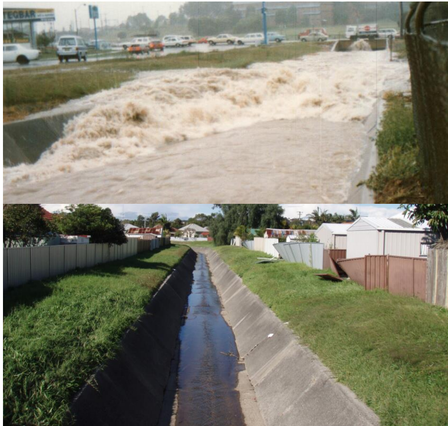
Figure 6. Fast-Flowing Concrete Open Channel in Throsby Creek Catchment (Top image courtesy of David Gibbins)
